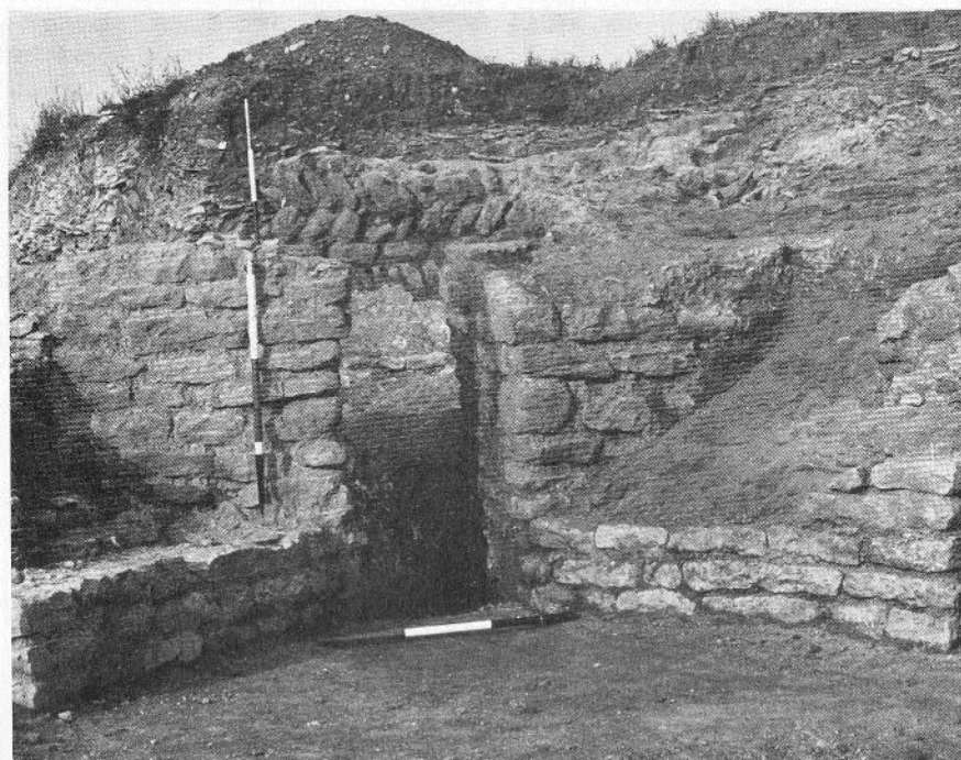
Fig 18 The Helpston limekiln
